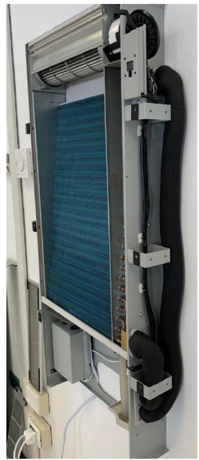
PUT INSULATION IN ALL THE EXTERNAL PIPE
