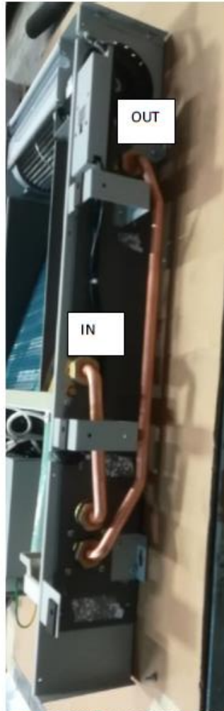
PIPE CONNECTION WITHOUT INSULATION
