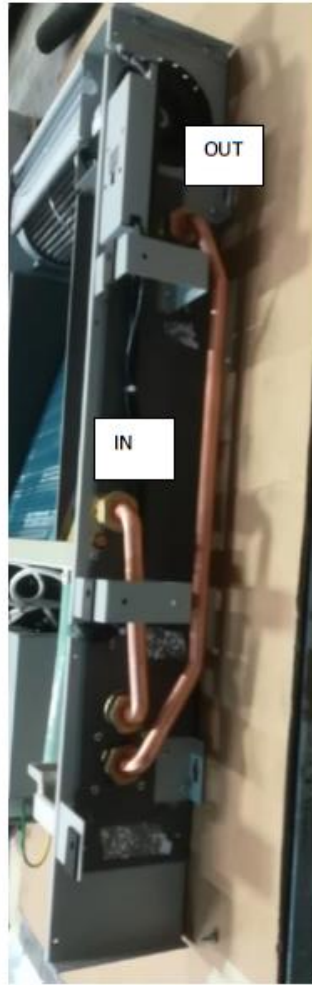
PIPE CONNECTION WITHOUT INSULATION
