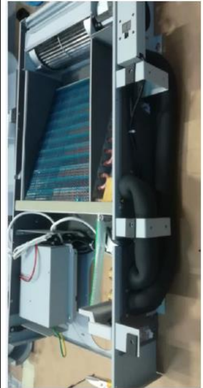
PUT INSULATION IN ALL THE EXTERNAL PIPE
