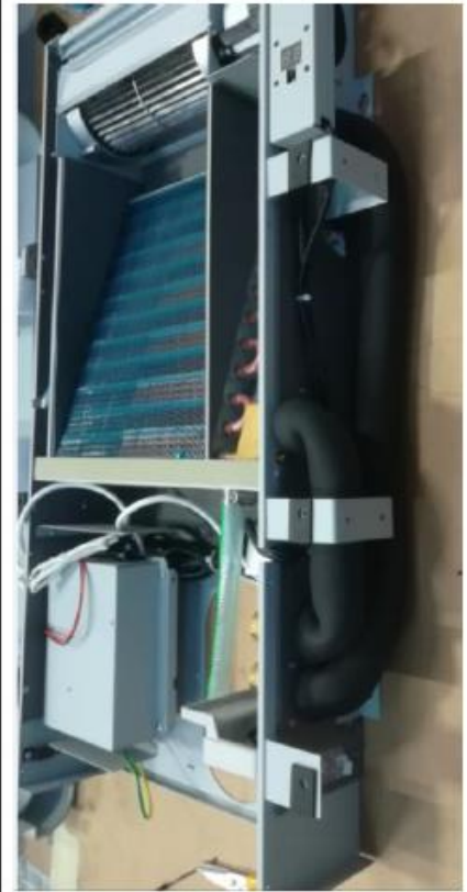
PUT INSULATION IN ALL THE EXTERNAL PIPE
